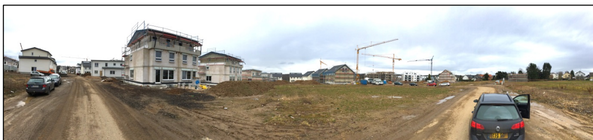
Fig.5 – Land re-allocation, Bonn – 186 Municipally-enabled serviced plots under construction.
